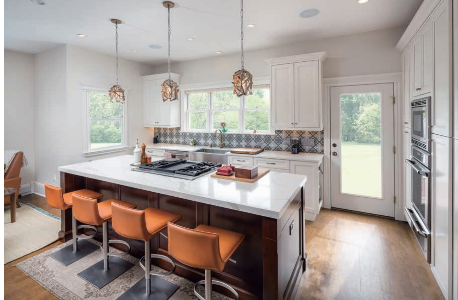
▲ The cabinet to the left of the exterior door was custom built with a false decorative panel on the front and an open side on the end for storage.
